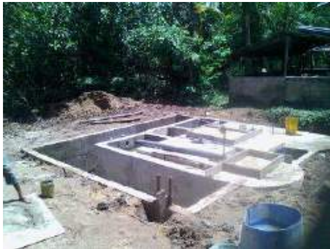
Medium scale biogas plant 15m 3 for farms in Ruwan Sampath's Piggery farm Welivita with the RDB loan scheme.
