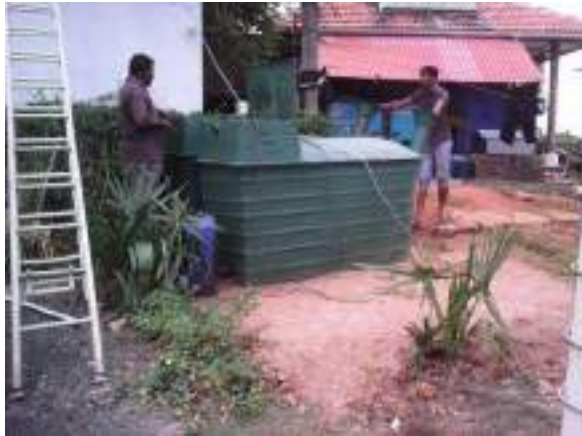
Domestic fiber glass biogas plant (design and manufactured under ETB logo)
