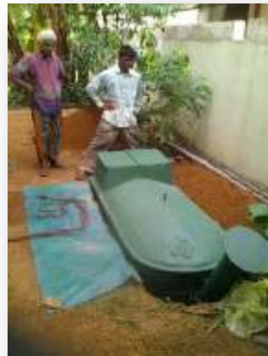
Domestic fiber glass biogas plant (design and manufactured under ETB logo)
